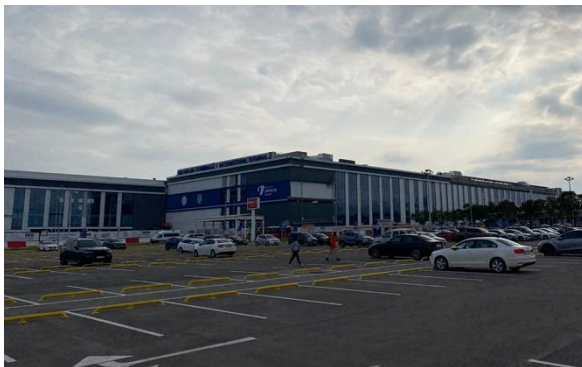
Figure 5 New Terminal 2 after Extension Works
